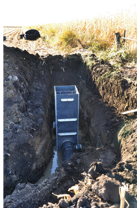
Figure 10. Drainage water management, also known as controlled drainage, uses a water control structure such as the one being installed at this site in Sac County, Iowa, to raise the depth of the drainage outlet, holding water in the field during periods when drainage is not needed. (Photo courtesy of Lynn Betts, National Resources Conservation Service [NRCS]/Soil and Water Conservation Society [SWCS].)
