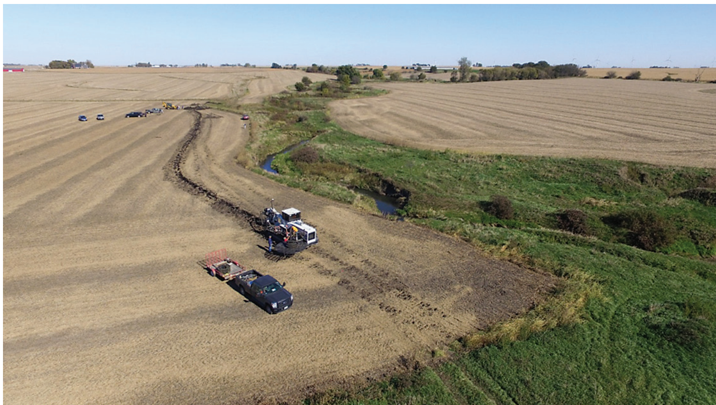
Figure 11. Saturated buffers divert tile drainage water into a shallow lateral pipeline distributed parallel to a water body, as shown in this installation in Story County, Iowa, to raise the water table within the buffer and enhance nutrient uptake by plants while slowing subsurface water outflow into the adjacent stream. (Photo courtesy of Lynn Betts, NRCS/SWCS.)
