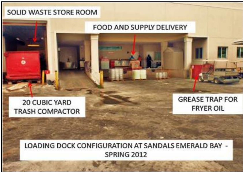
17.2 Visual illustrating the location of the trash compactor in relation to the food and supply delivery station for Sandals Emerald Bay. The unsorted trash adjacent to the food loading dock creates challenges with food safety and hygiene
