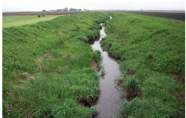
Figure 4.3. Typical headwater stream or ditch in the glaciated, agricultural landscape of the upper Midwest. Such streams and ditches are periodically dredged to ensure drainage of the landscape during wet periods. (Photo courtesy of Todd Royer.)
