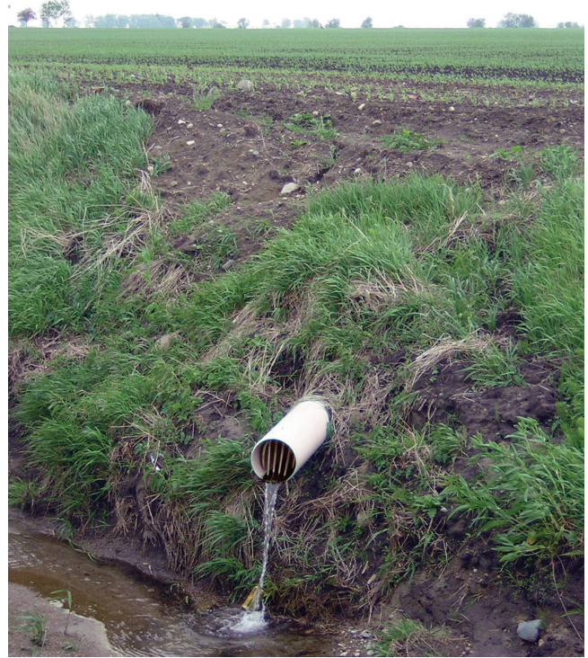
Figure 3.3. Typical tile drain outlet discharging to a headwater stream or ditch. Tile drainage is common in the upper Midwest, where poorly drained soils and low topographic relief necessitate artificial drainage of wetlands and mesic prairie when the land is farmed. (Photo courtesy of Todd Royer.)
