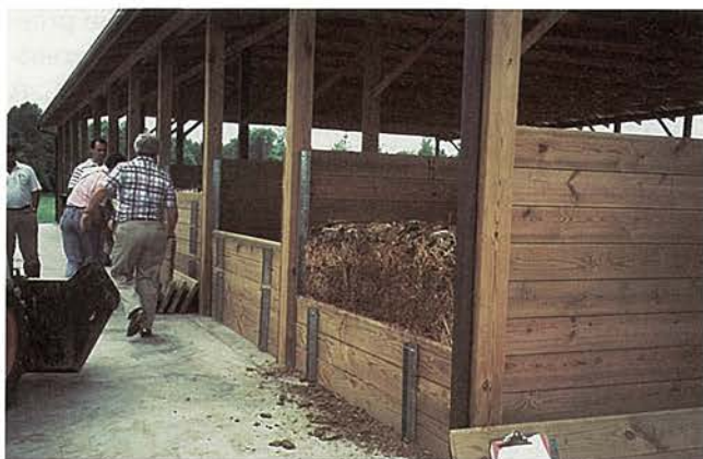
Figure 4.2. Poultry mortality composting building showing the initial compost bin prior to movement of the compost into the secondary bin. Photograph courtesy of Gerald B. Havenstein, Department of Poultry Science, North Carolina State University, Raleigh.
