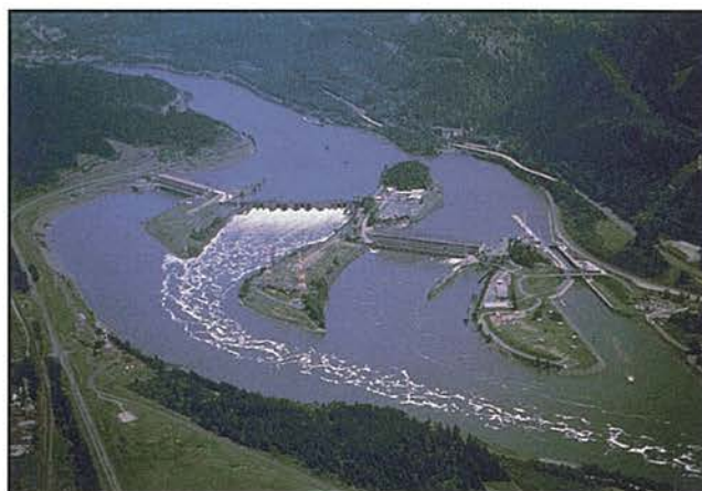
Figure 5.4. Bonneville Dam and Power Plant on the Lower Columbia River. Photo courtesy of the U.S. Army Corps of Engineers.
