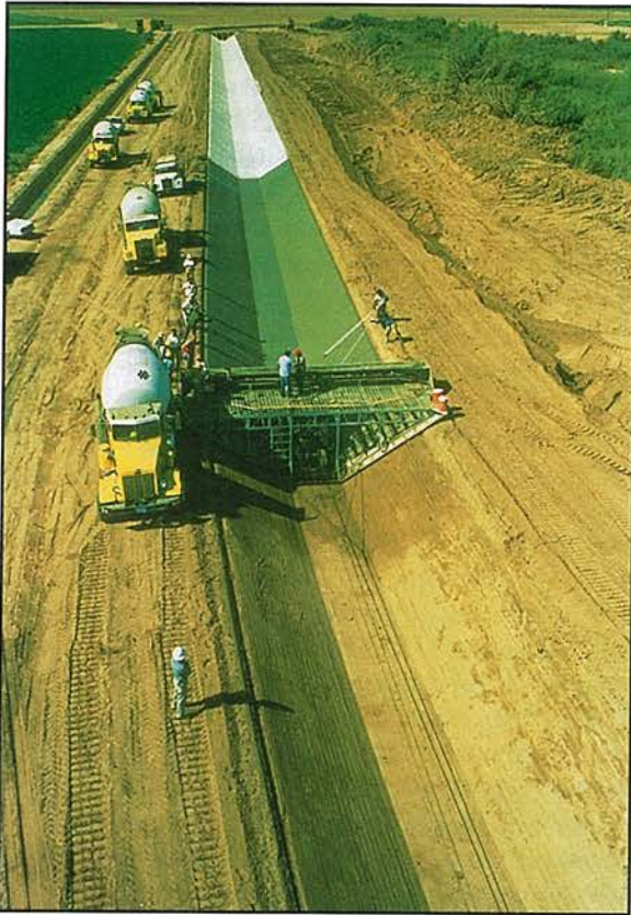
Figure 5.26. Irrigation canal lining in the Imperial Valley. Photo courtesy of the Imperial Irrigation District.
