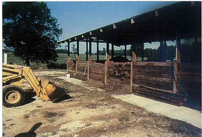
Figure 6.1. Roofed composter for dead animals, with concrete floor, wood bin walls and roof overhang to protect the work area. Photograph courtesy of Alan L. Sutton, Purdue University, West Lafayette, Indiana.
