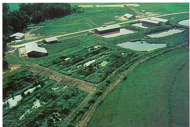
Figure 3.4. Aerial view of constructed wetlands treating swine lagoon effluent. Photograph courtesy of Thomas A. McCaskey, Auburn University, Auburn, Alabama.
