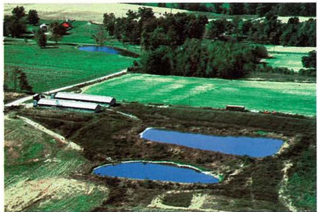
Figure 3.2. Two-stage lagoon with recycled water for swine manure collection, storage and treatment. Photograph courtesy of Don D. Jones, Purdue University, West Lafayette, Indiana.
