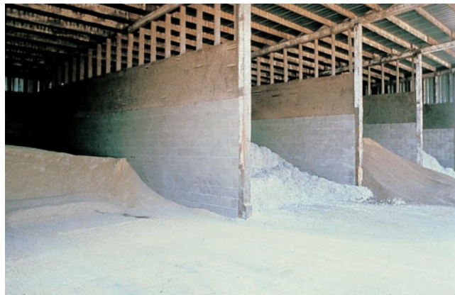
Figure 4.31. Commodity barn, California dairy. Whole cottonseed in center bay. Photograph courtesy of Thomas Shultz, University of California, Cooperative Extension, Tulare, California.
