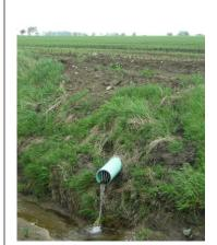
Typical tile drain outlet discharging to a headwater stream or ditch.
